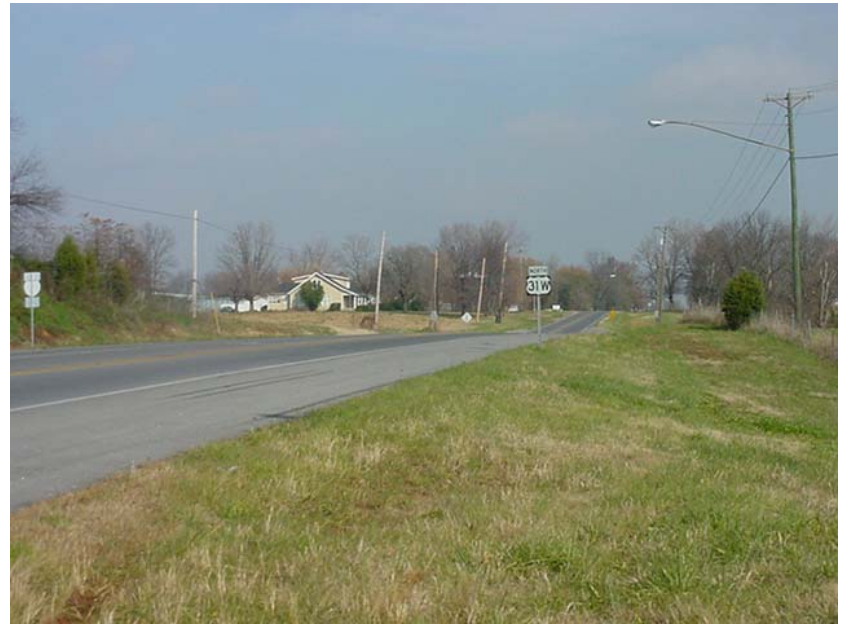
US 31W north of northeast KY 1008 (looking north)
