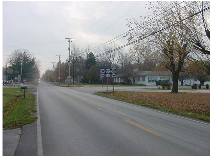
Intersection of KY 100 and southwest KY 1008 (looking east)
